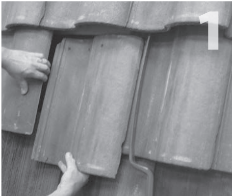
1 Remove tile at selected location of mount.
