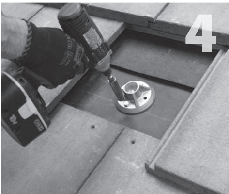
4 Align QBase over rafter center and drill two 7/32" pilot holes. Place grade-8 machine bolt under QBase in hex slot, threads pointing up. Lag QBase into rafter on marks.
