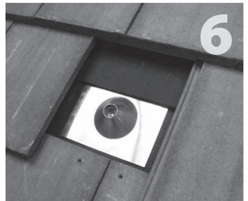
6 Take care to do a quality installation. When using the paper method, cut a piece of paper 18" wide to slide under the course above, and over the primary flashing of the mount. See reverse side for details on the three-course method.
