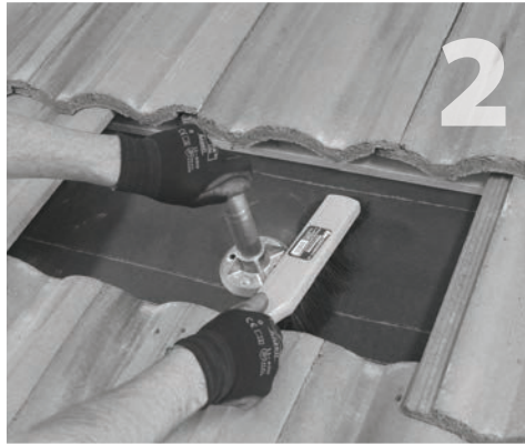
Clean away dust and debris around QBBase.
