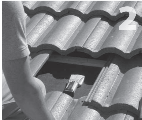
2 Locate and mark center of rafter.
