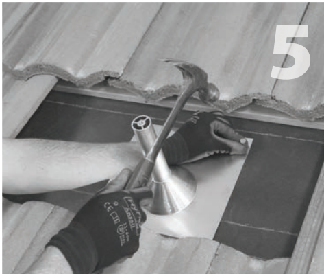
Fasten the sub-flashing into place with two roofing nails, one in each top corner.
