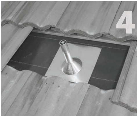
Install the sub-flashing over the post, making sure the edge closest to the cone is on the downhill side.
